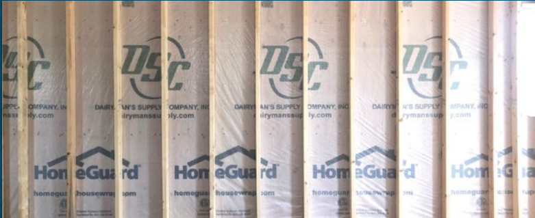
House Wrap Vapor Barrier Recommended if you plan to insulate
