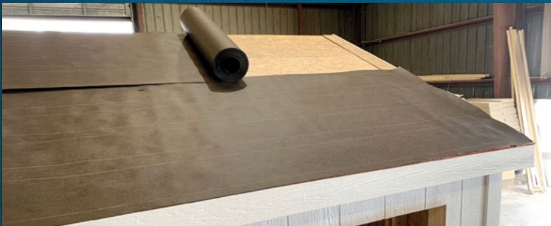
Tar Paper Under Roofing Only Recommended for Shingle Roofs
