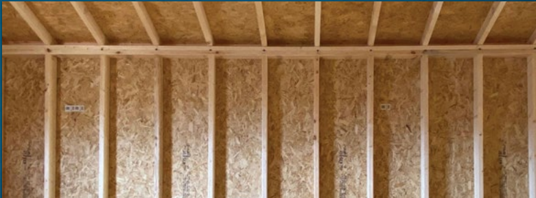
For Buildings with Painted LP Smart Panel Upgrade to 16" On-Center Trusses. Standard is 16" On-Center Studs and 24" On-Center Trusses.
